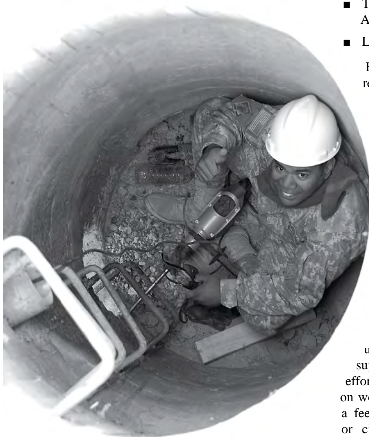
A Soldier modifies a manhole to add to an existing drainage system to accommodate the COB's expanding needs.
