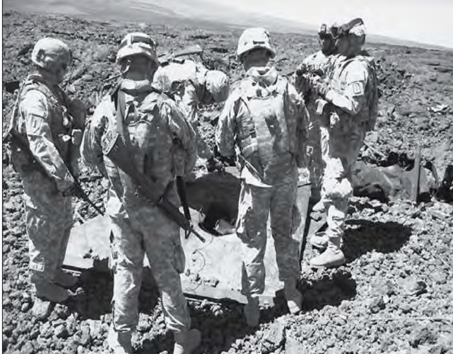
Sappers from the 65th Engineer Battalion conduct demolition operations at Pohakuloa Training Area, Hawaii.
