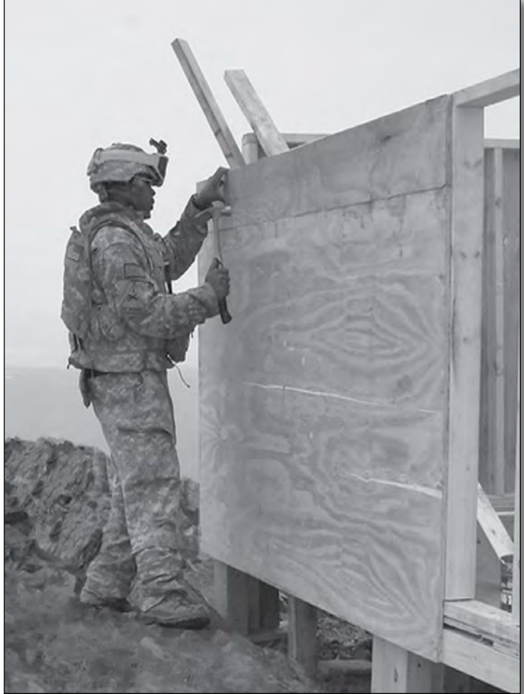
A Soldier from Bravo Company, 864th Engineer Battalion, Fort Lewis, Washington, nails the wall for a bunker at an outpost on an Afghanistan mountain.
