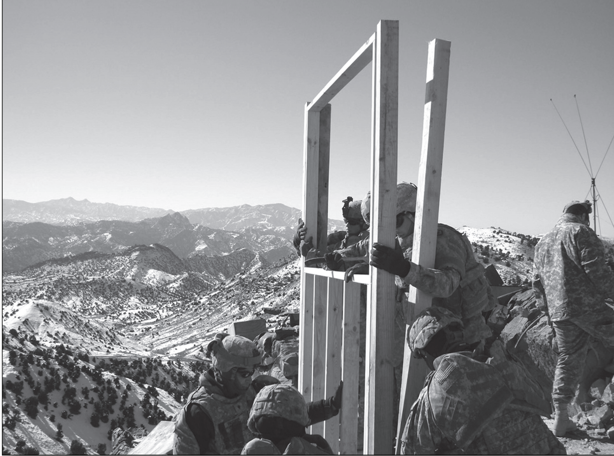
Engineers from Bravo Company, 864th Engineer Battalion, Fort Lewis, Washington, put up wall structures for a new bunker that will serve as an outpost in the middle of the mountains in eastern Afghanistan.
