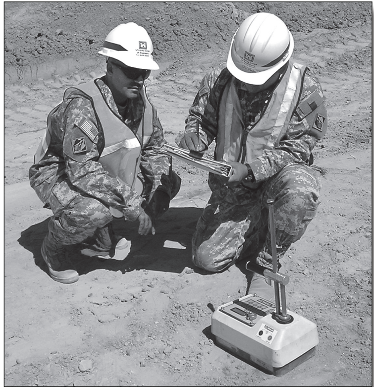
Soldiers use a nuclear densimeter to determine soil compaction and moisture content.
