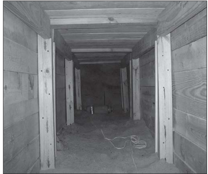
Figure 3. A look down the tunnel to the working face.
