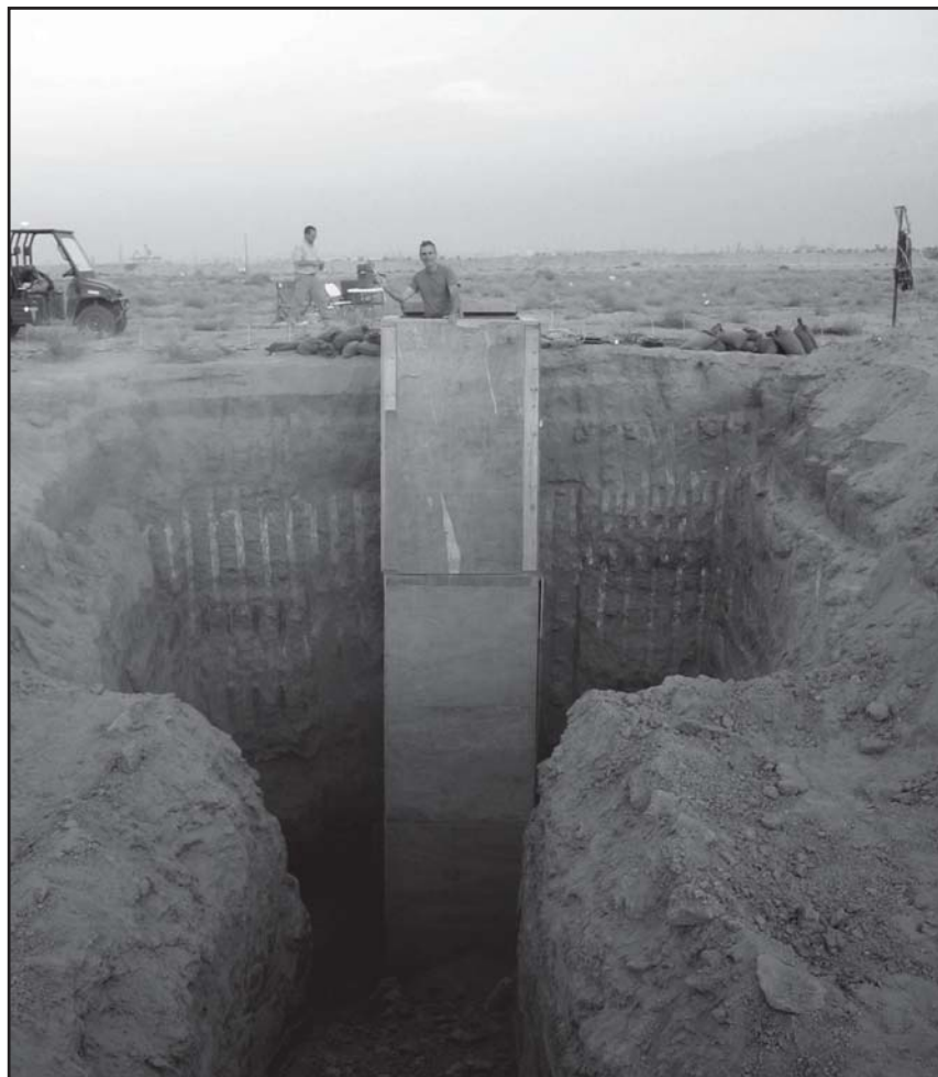
Figure 2. The shaft in place. Note the various layers of compacted silt.
