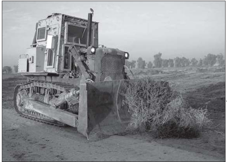
A D7 bulldozer grubs the project site.
