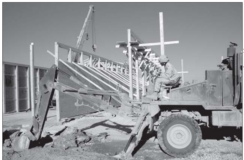
A small emplacement excavator (SEE) operator digs through the rocky terrain so sewage pipes can be laid.
