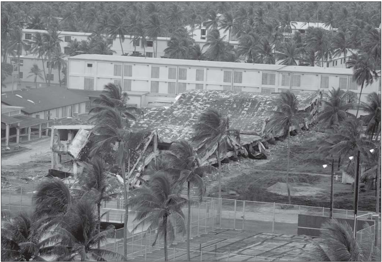
The building was reduced by at least half by the blast.
