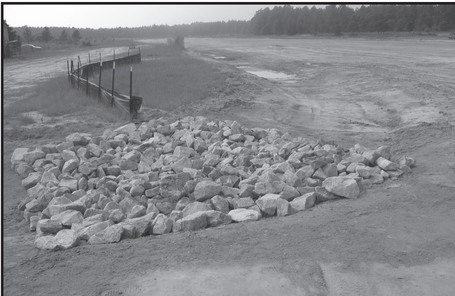
Drainage swale and check-dams provide drainage for the landing zone.
