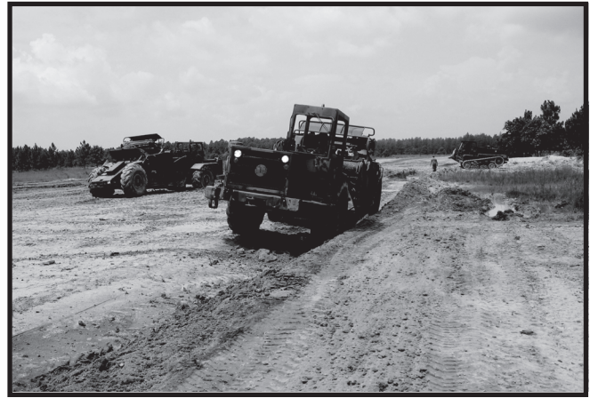
Grading, leveling, and drainage construction operations using the 613BS Scraper and DEUCE
