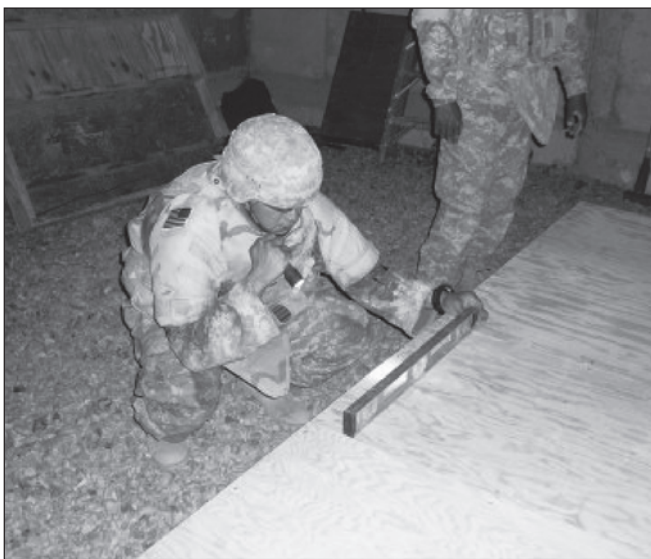
A Soldier ensures that the building floor is level.
