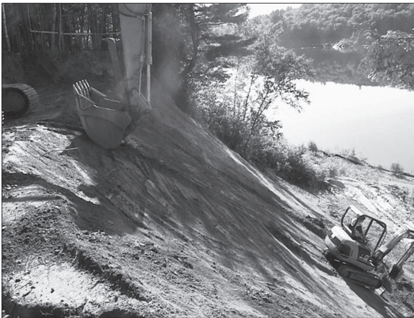
The slope was regraded prior to placing riprap for stabilization.
