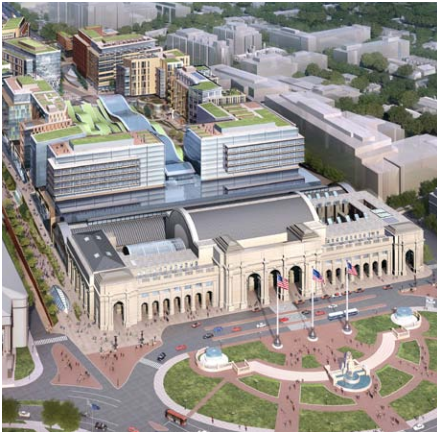
View of the historic station, train shed and air rights development from the southwest. Image courtesy of Akridge/SBA.
