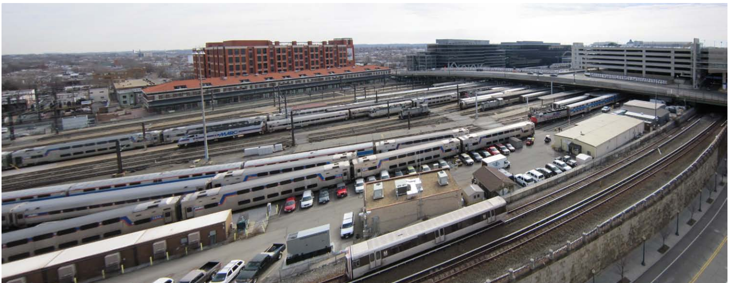
View of station looking southeast showing midday storage of equipment on active platforms
