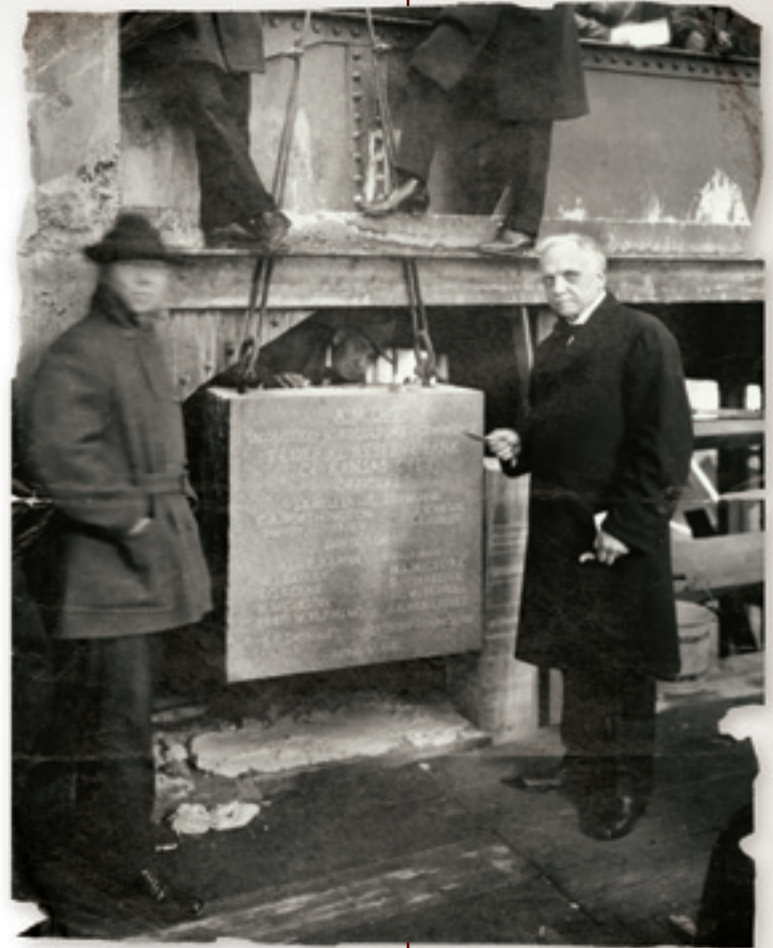
Federal Reserve Bank of Kansas City Gov. Jo Zach Miller, Jr., during the cornerstone ceremony at the Bank’s headquarters building, April 16, 1921.
