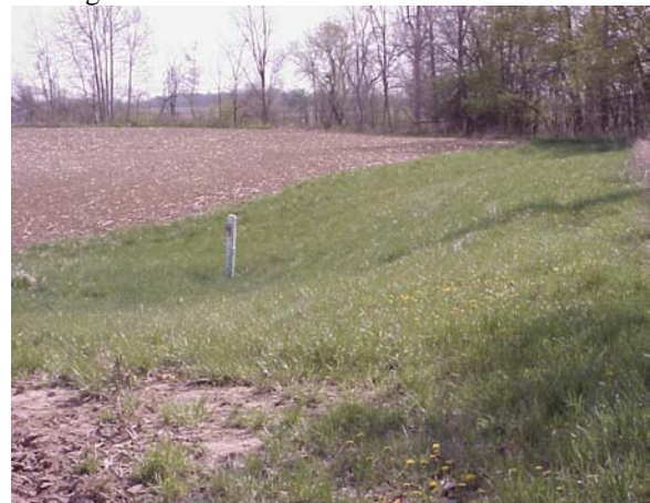
WASCOB embankment (right) and riser for drainage
