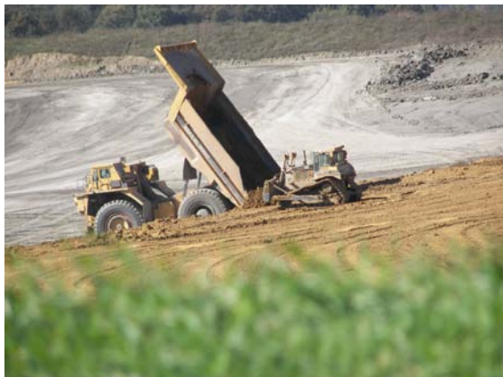
Soil material being replaced over graded spoil as part of the land reclamation process. Photo courtesy of Peabody Coal
