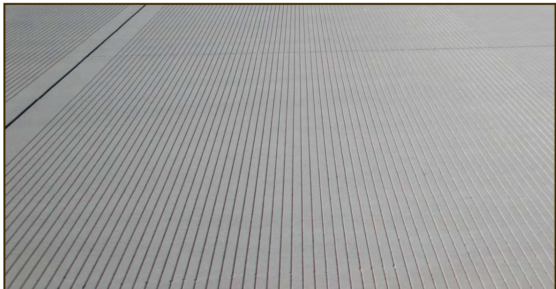
Runway Grooving (Friction Treatment)
