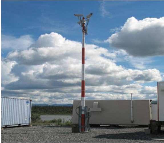
Figure 6-34. Weather Camera (WCAM) pole
