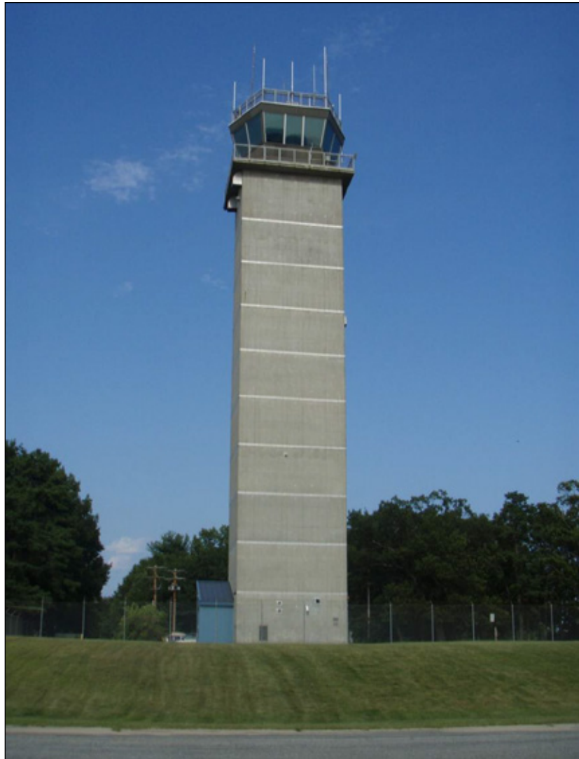
Figure 6-3. Airport Traffic Control Tower (ATCT) facility
