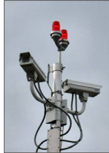
Figure 6-34. Weather Camera (WCAM) pole
