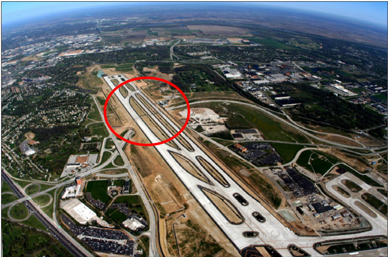
Figure 7-1. Tunnel under a runway and parallel taxiway
