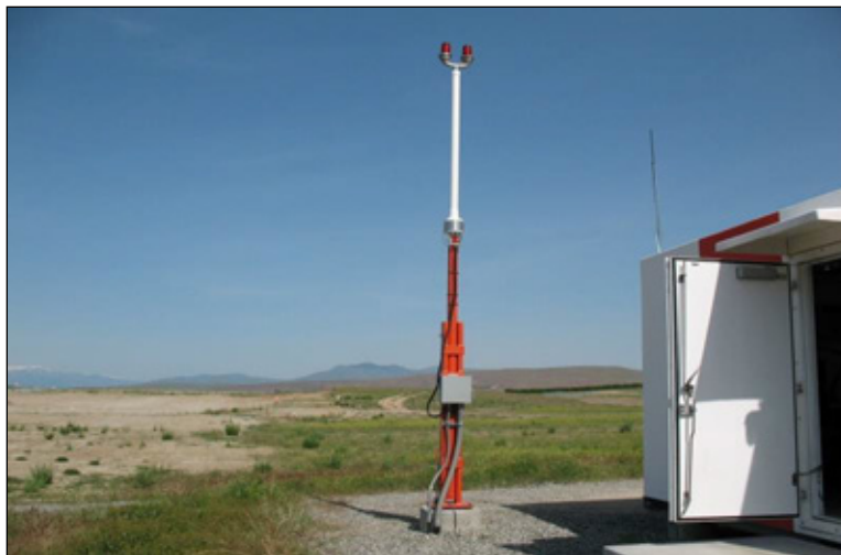
Figure 6-25. Distance Measuring Equipment (DME) antenna
