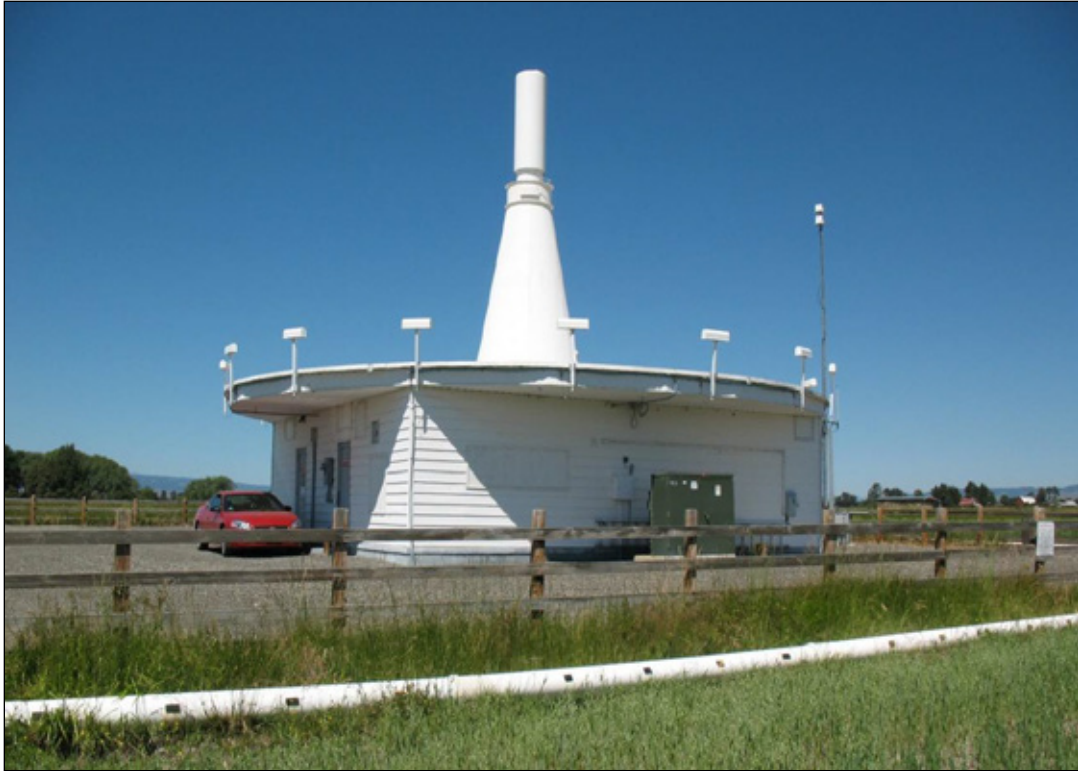
Figure 6-27. Enroute VHF Omnidirectional Range (VOR) facility
