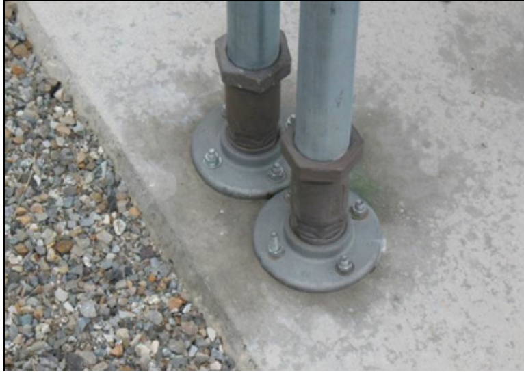
Figure 6-2. Two frangible connections
