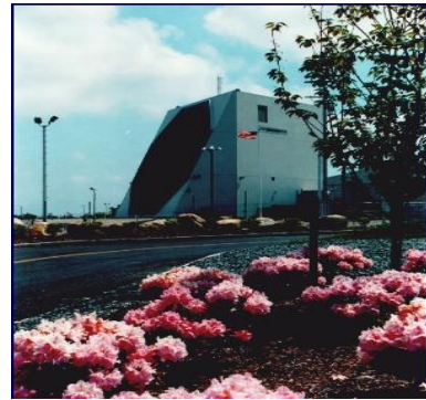
AFSPC PAVE PAWS Radar Cape Cod Air Force Station
