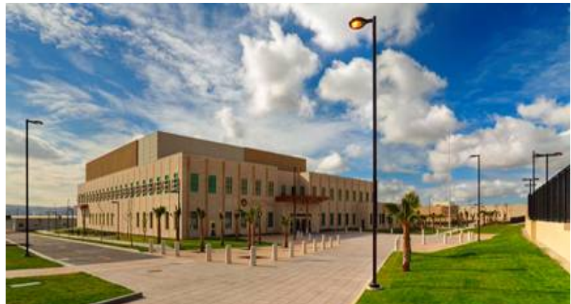
U.S. Consulate General Tijuana Building at new location in Mesa de Otay Source: U.S. Department of State
