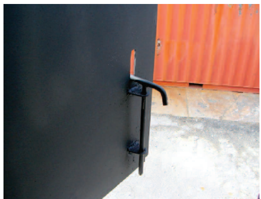
Figure C-6: Window & Latch Construction
