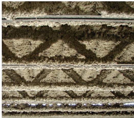
Figure C-4: Fireproofing added to structural steel
