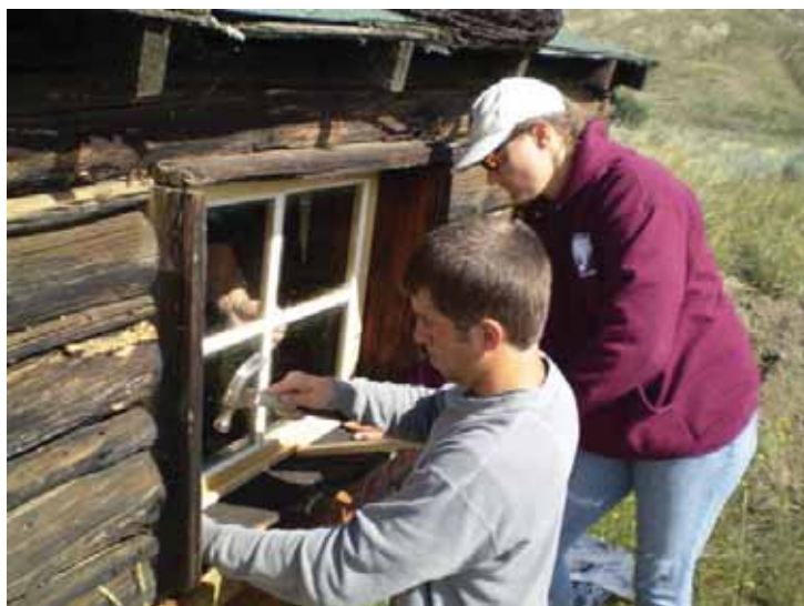
Stabilization work at the Hagadone homestead.
