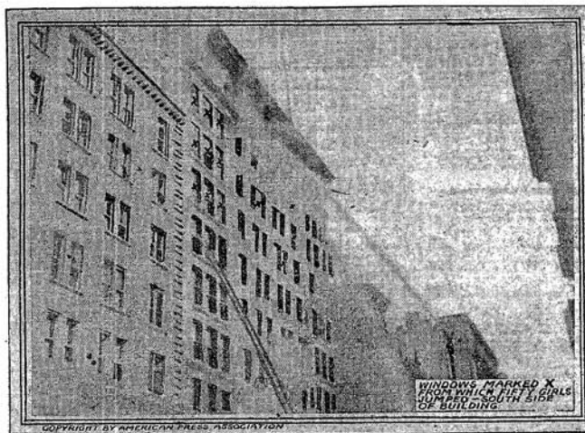
The Burning Building at 23 Washington Place.
