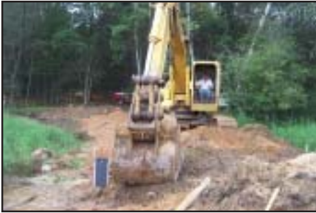
Restoring a wetland by constructing a berm
