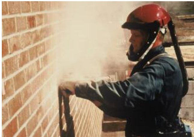
Grinders who perform tuckpointing without dust controls are frequently exposed to extremely high silica levels. (Photo courtesy of CPWR.)
