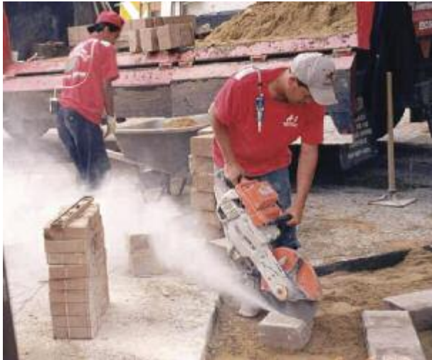
Employee operating a handheld masonry saw without the use of appropriate dust controls. (Photo courtesy of OSHA.)
