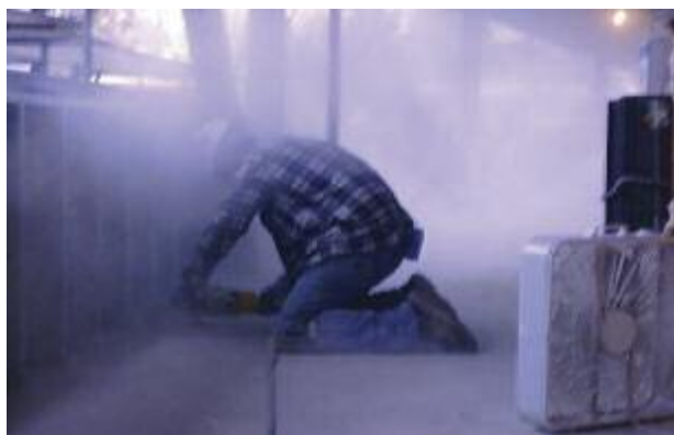
Using a grinder in poorly controlled conditions. (Photo courtesy of the University of Washington.)
