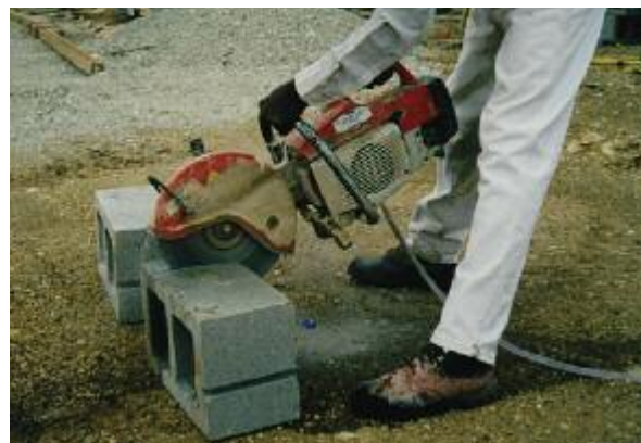
When applying water to the blade, exposures of handheld saw operators to silica are considerably reduced. (Photo courtesy of OSHA.)
