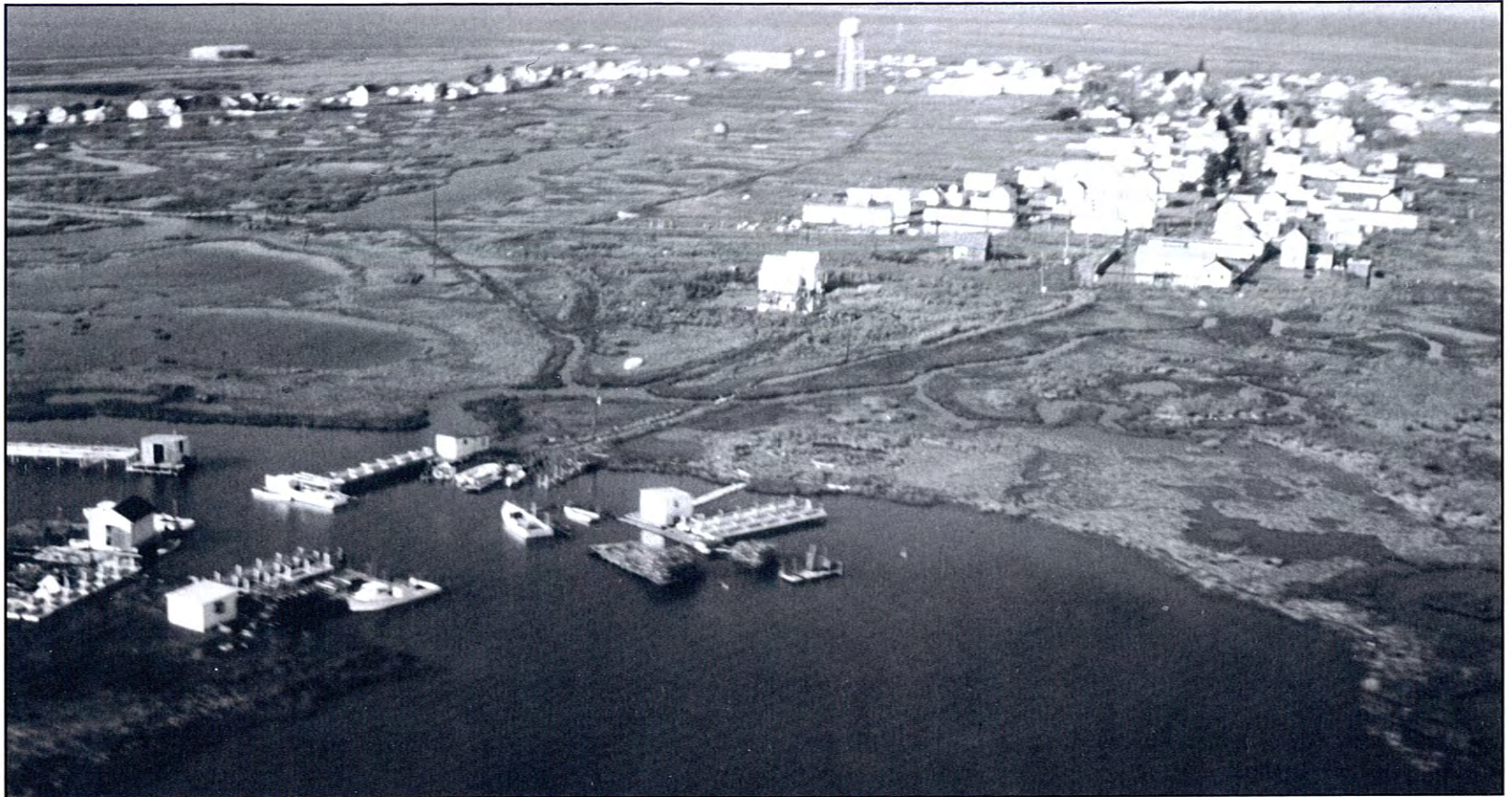
Figure 35. The towns on Smith Island exhibit low relief and therefore much vulnerability to even small increases in sea level (USFWS photo).
