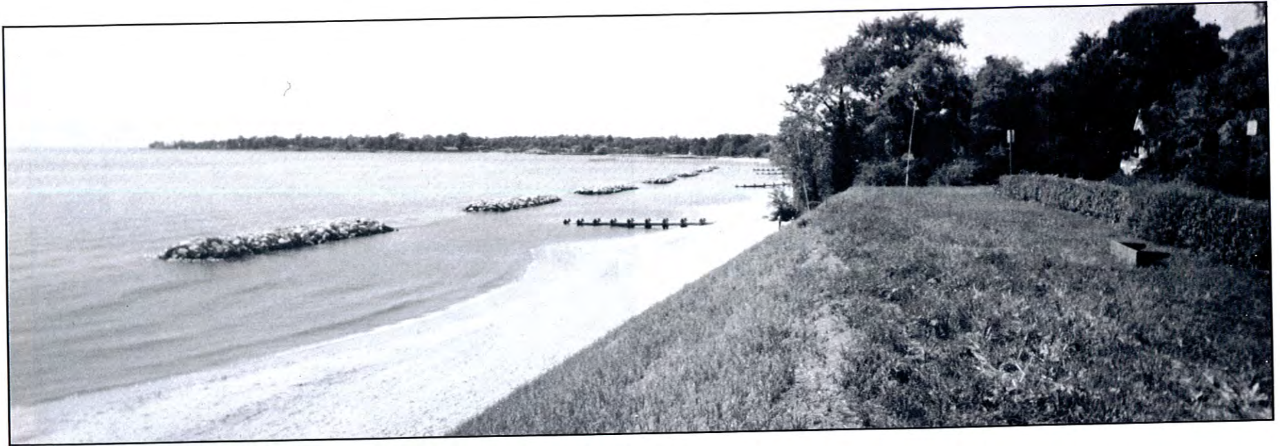
Figure 39. Offshore breakwaters with beach fill have been used at Bay Ridge, Annapolis to protect the cliff and provide a recreational beach (photo by Ed Fulford).
