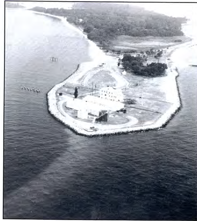
Figure 27. The Point Lookout Lighthouse area has been restored and stabilized but at the expense of the "point" (see Figure 26) (photo by Steven Leatherman).
