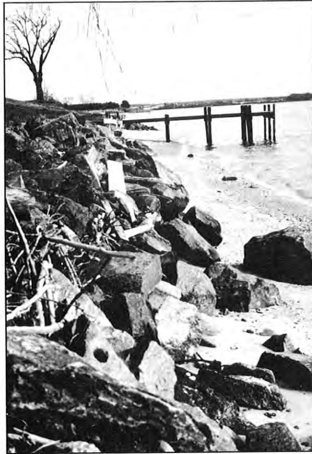
Figure 17. Structurally stabilized shores in the Bay provide no place for marshes to form or migrate (USFWS photo).
