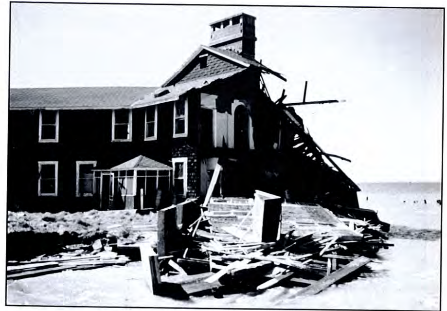
Figure 40. A hunting lodge on Barren Island collapses as shore erosion continues unabated (USFWS photo).
