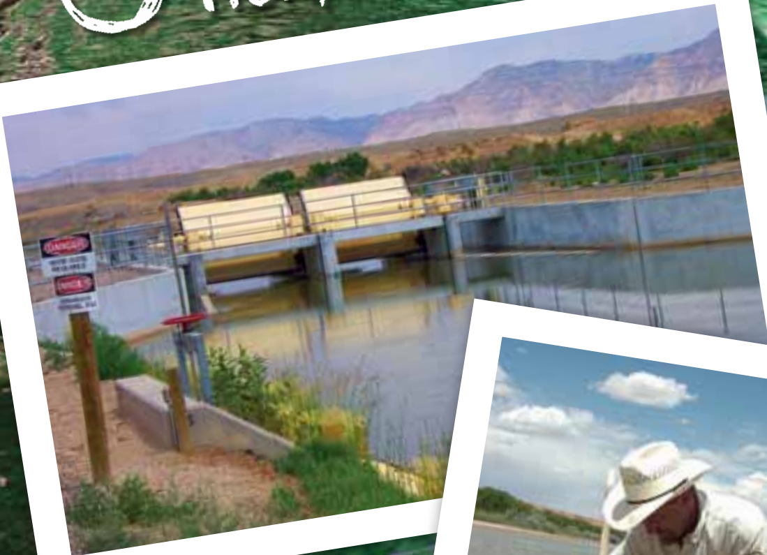
(Above): Check structures constructed at the privately owned Grand Valley Irrigation Project in western Colorado reduce water diversions by 6 to 34 percent each year while meeting irrigation demands. The conserved water benefits endangered fish in the Colorado River.
