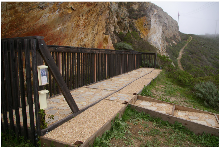
In FY 2008 VAFB completed refurbishment of a rock art viewing platform for easier and safer visitation by Chumash Tribal Elders and the many visitors to Honda Ridge rock art site. Following consultation with the Tribe, upgrades were completed to the platform, enhancing the setting of this sacred site. A guest register, interpretive panel, and pamphlet dispenser at the trailhead help foster respectful visitation by the public.
