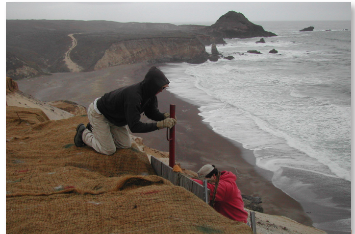
Not your typical Section 110 management practice: stabilizing 9,000 year old shell midden using bio-degradable erosion control fabric. Native wind-tolerant plants were added to the fabric to trap wind blown sand. One year later, much of the fabric is buried by sand, and new plants are naturally establishing.
