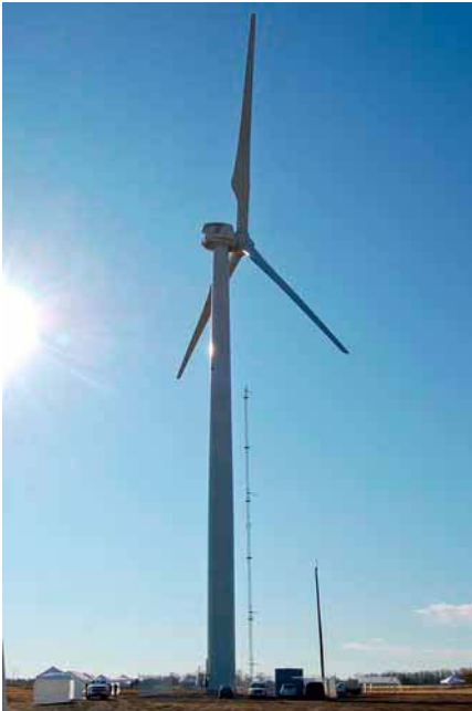
Utility-Scale Wind turbine with an anemometer tower in the background. Credit: University of Minnesota College of Science and Engineering
