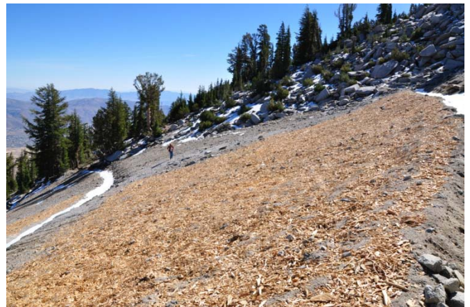
Figure 2: Section of Upper Bonanza Run amended with wood chips
