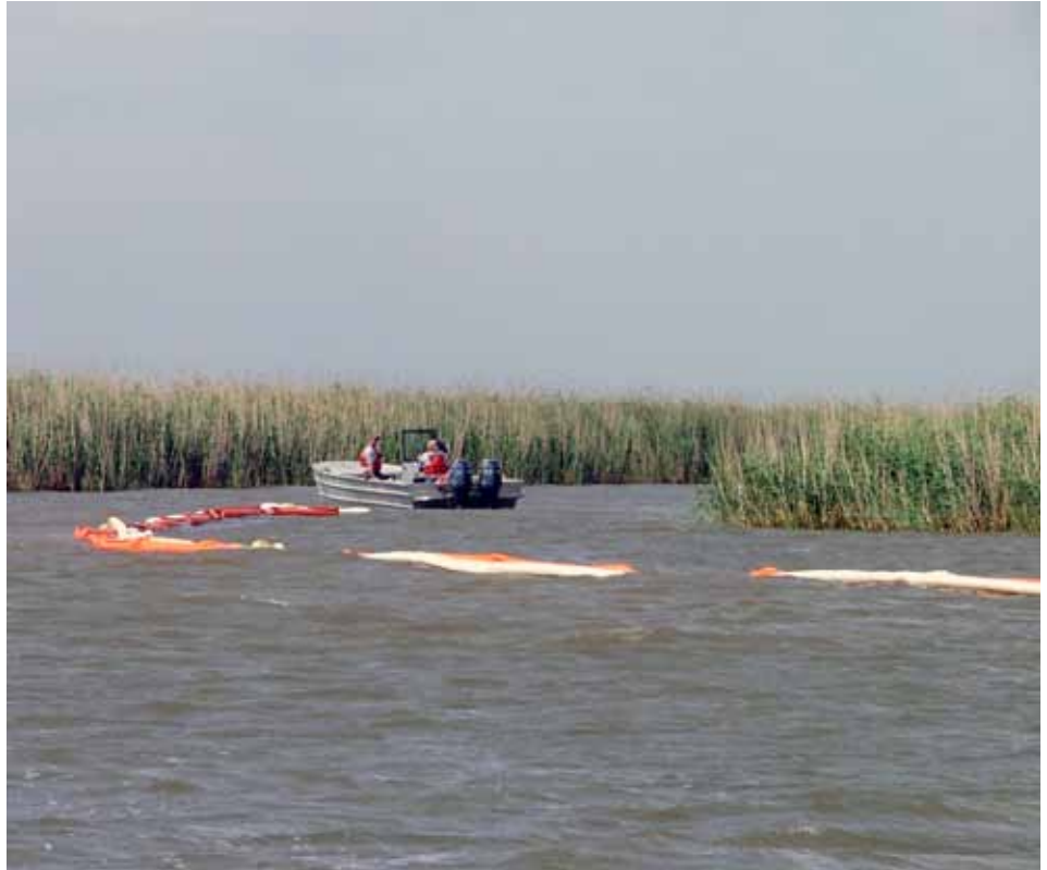
Hard boom and absorbent boom require frequent monitoring to ensure effectiveness, photo by USFWS/Drew Wirwa.
