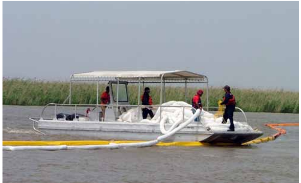
Workers place absorbent boom on Delta NWR, photo by USFWS/Drew Wirwa.
