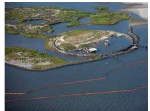
Containment boom is staged at the Breton National Wildlife Refuge.
