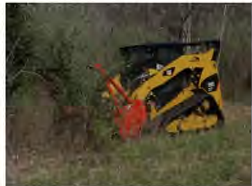
NNIS-IDIQ contractor performing autumn olive control using skid-steer and drum cutter/mulcher
