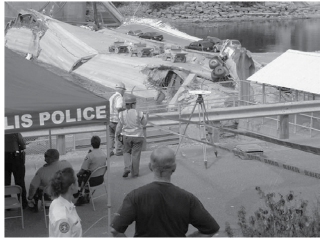
Minnesota OSHA investigators set up a safety perimeter around the site of the bridge collapse.
