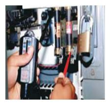
Worker was performing testing on the circuit without PPE.
