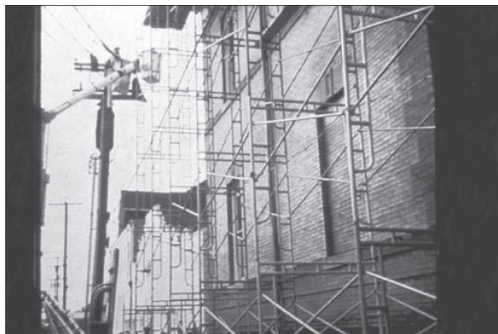
This power company worker is placing insulated sleeves ("eels") over the power line in this photo.
