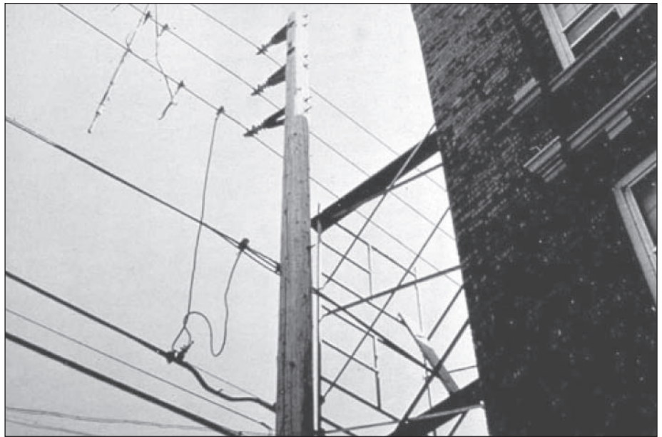
This scaffold has been protected from electrical hazards: three power lines at the top have been de-energized, jumpered together and then electrically grounded by the power company.
