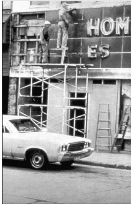
He's standing on a sawhorse, placed on top of a scaffold, and has no fall protection...
