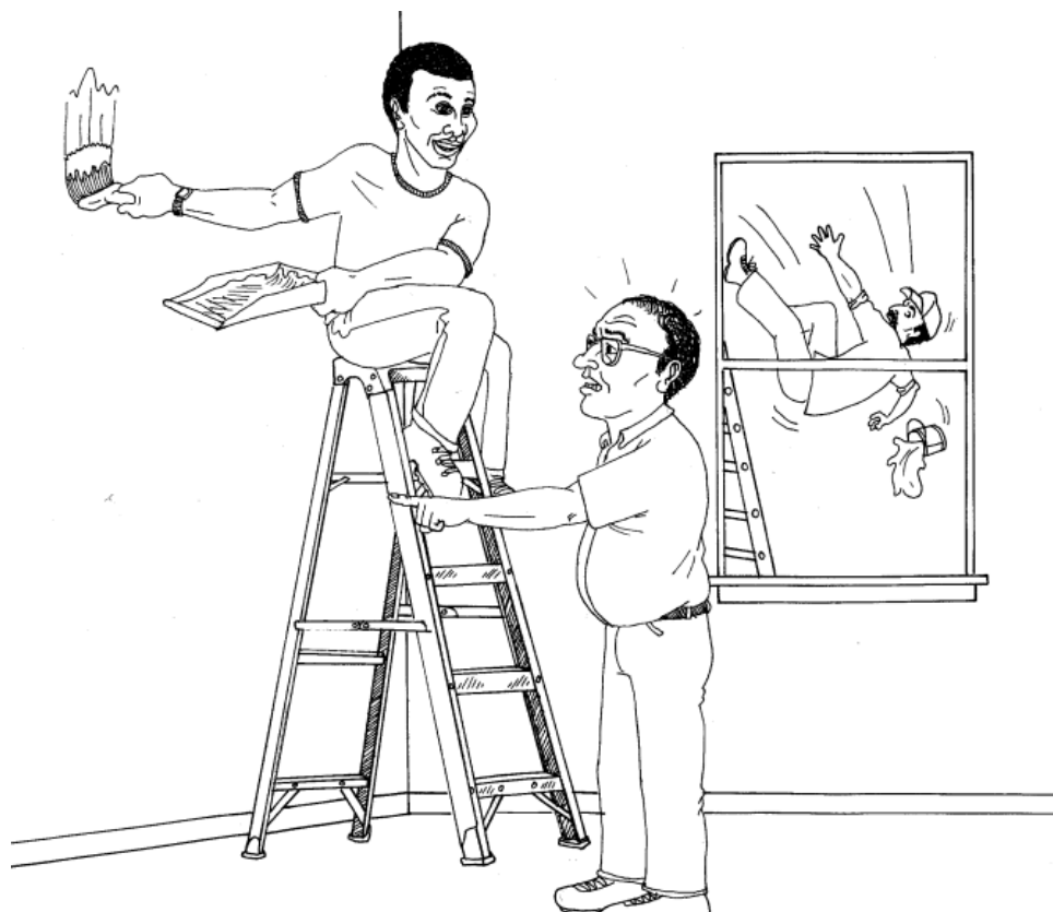
Unsafe Work: List the safety hazards inside and outside of the building.
