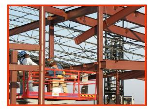
All materials being lifted must be picked up evenly so they don't shift causing part or all of the load to fall. Be sure to properly secure the load and don't lift more than the equipment can handle.
