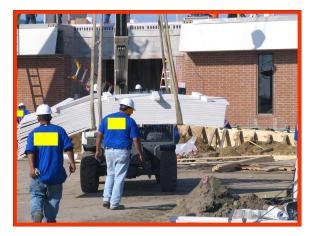
The disadvantages of using heavy equipment are that they are dangerous and often the operators have a limited view. If you are in a position where the operator cannot see you, your very life is in danger. Many workers have been struck and then run over by heavy equipment.
