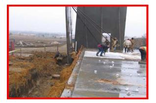
When placing pre-fabricated walls or forms, ensure that all panels or structures are properly braced and supported to keep the wall or form from toppling over and causing severe injury or death to workers.
