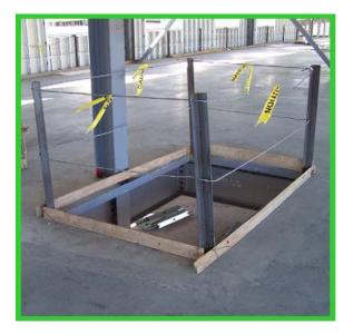
Steel banding and plastic banding <u>shall</u> <u>not</u> be used as top rails or midrails. {see 1926.502(b)(8)}
