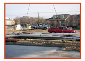
Remember, the load must be lifted with the hook over its center of gravity. To make a level lift, the hook must be directly above this point. If the hook is too far to one side of the center of gravity, dangerous tilting will result causing unequal stresses in the different sling legs.
