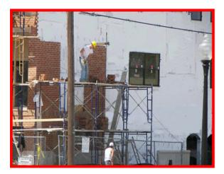
When you work or walk below elevated work surfaces, you may be exposed to falling objects. Falling objects may strike you on the head or any other part of your body. These falling objects are the primary reason you need to wear a hardhat.
