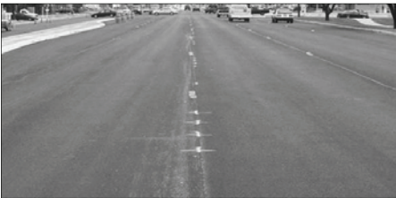
Temporary pavement markings should not be in place more than 2 weeks unless justified using engineering judgment.
