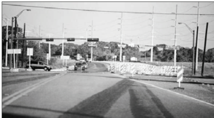
If no longer applicable, pavement markings shall be removed or obliterated in long-term work zones.
