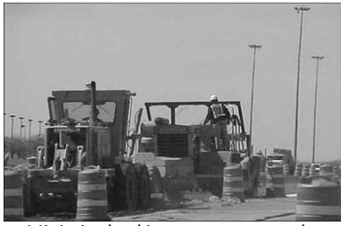
Minimize backing-up maneuvers by construction vehicles
