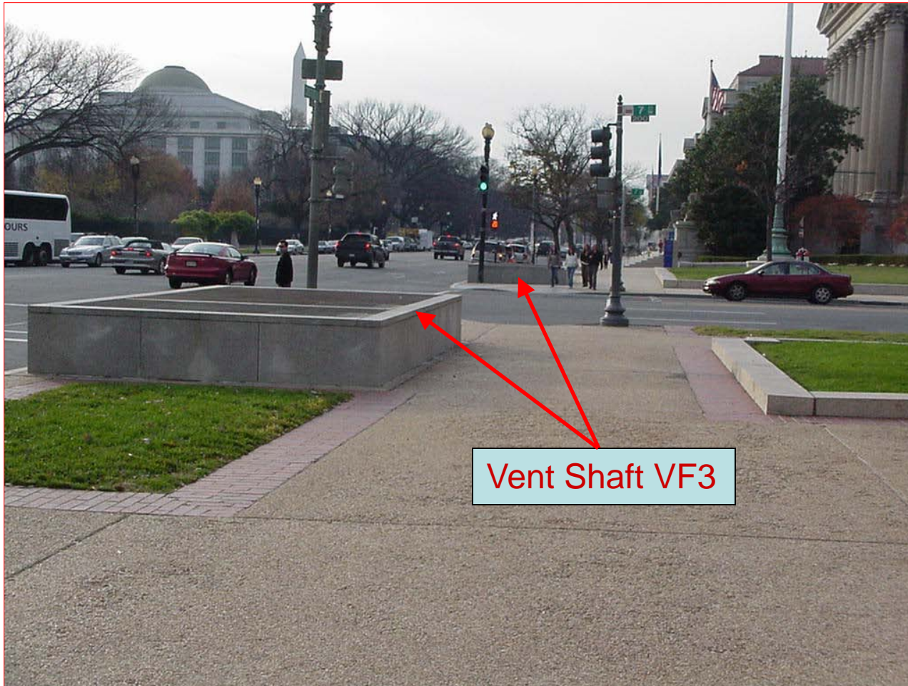
Vent Shaft VF3 – 701 Constitution Avenue, N.W.
