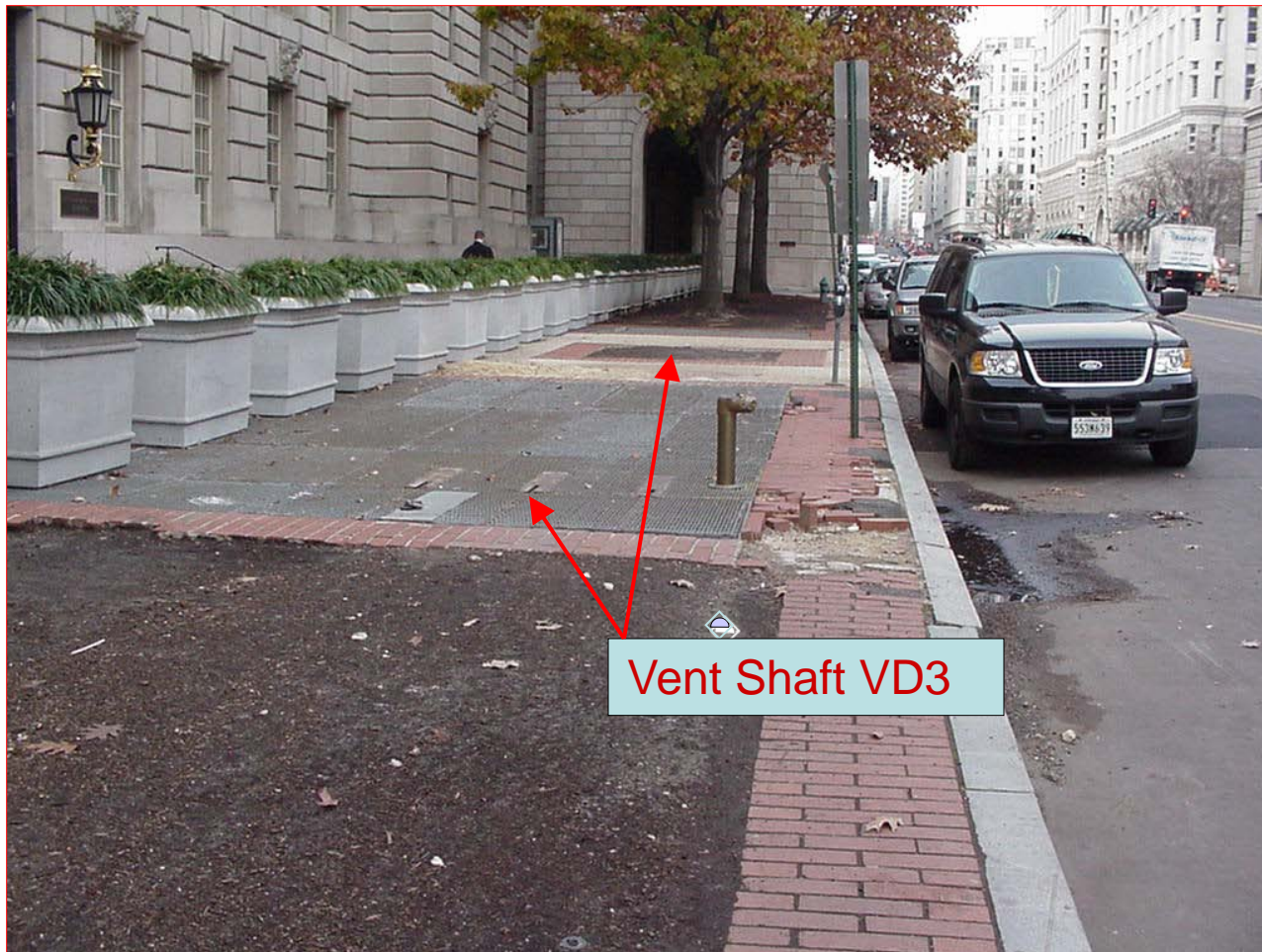
Vent Shaft VD3 - 310 12th Street, N.W. – Existing Condition
