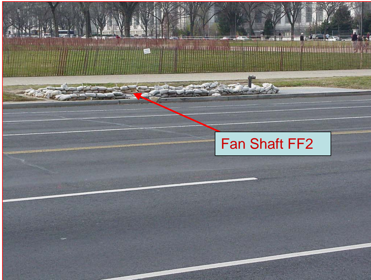
Fan Shaft FF2 – 1 7 th Street, N.W.
