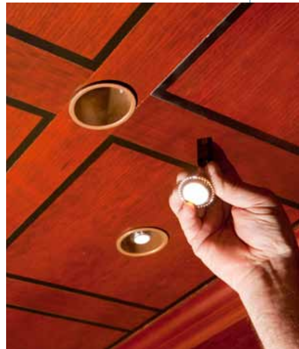
LED lighting is retrofit to provide a more energy-efficient alternative.
