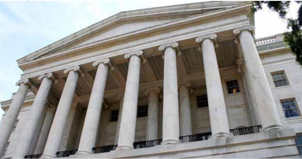
A view of the front portico of the Longworth House Office Building.
