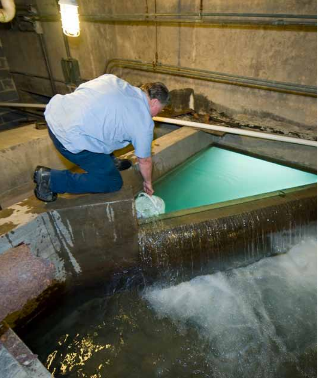
An employee tests water quality in a fountain filtration system.
