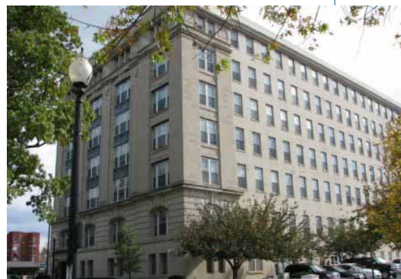
The Eney, Chestnut, Gibson Memorial Building is the home of the Capitol Police Headquarters.
