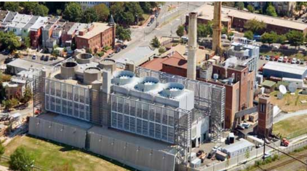
The Capitol Power Plant celebrated its centennial in FY 2010.
