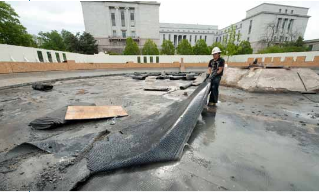
Construction in progress during the Bartholdi Fountain Renovation.
