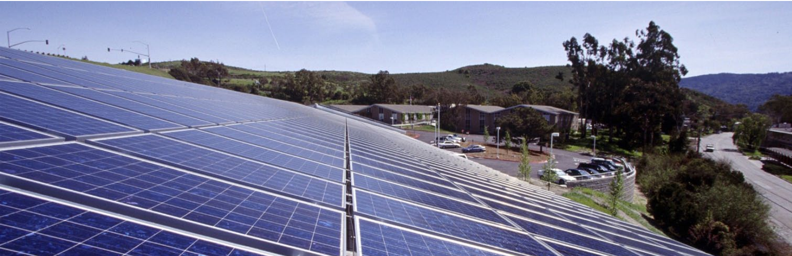
"San Mateo County Sheriff's Forensic Laboratory and Coroner's Office, San Mateo, California." Photo courtesy of HOK.
