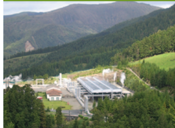
"Geothermal Power Plant, São Miguel Island, Azores, Portugal." Photo credit: Jonathan Herz
