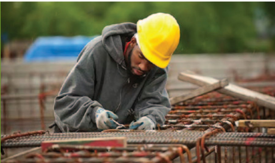
"Construction Training at The Challenge Program." Photo Credit: ChallengeProgram.org
