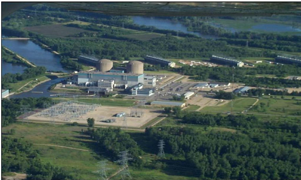
Prairie Island Nuclear Generating Plant
