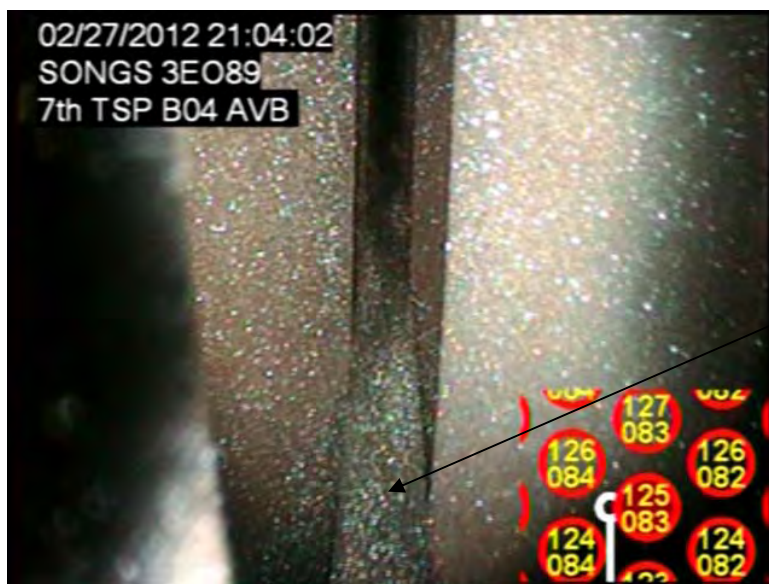
Photo-6 Tube Bundle Visual Inspection Image [Unit-3A]
