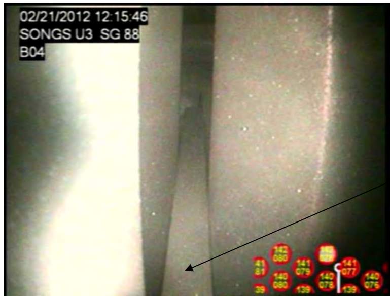
Photo-7 Visual Inspection Image of Outermost Tube Region [Unit-3B]
