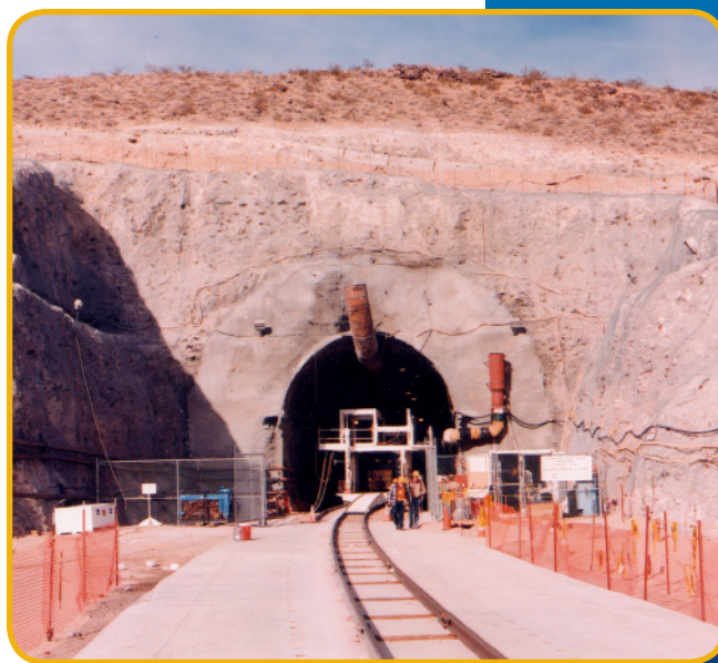
Yucca Mountain Tunnel Entrance
