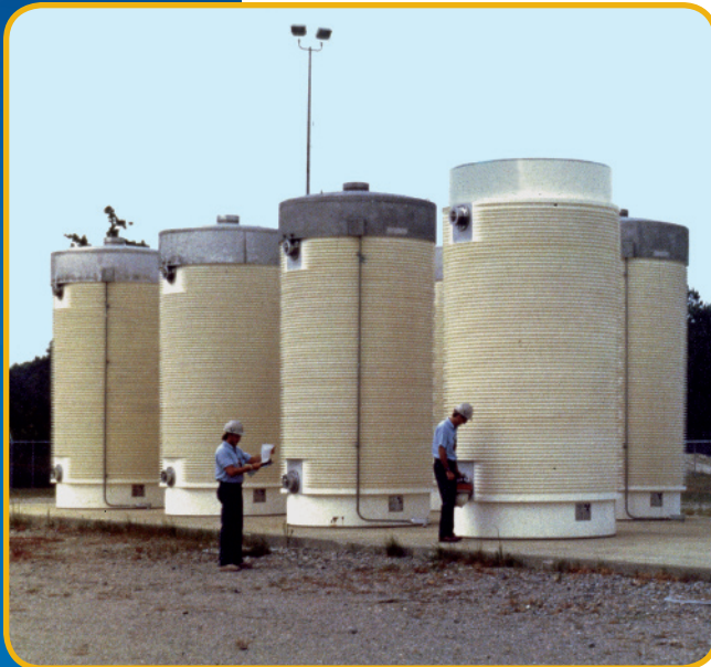
Dry Storage of Spent Fuel
