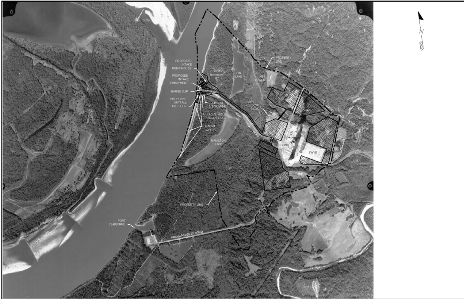
Figure 2-4. Aerial Photograph Depicting Grand Gulf Nuclear Station Unit 1 (November 21, 2001) and Construction Areas (Cross-Hatched Areas) for the Proposed Grand Gulf Early Site Permit Facility (SERI 2005, Figure 2.4-2)
