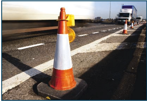
Highway work zone.
