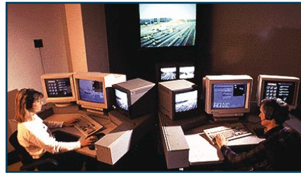
Traffic operations center.
