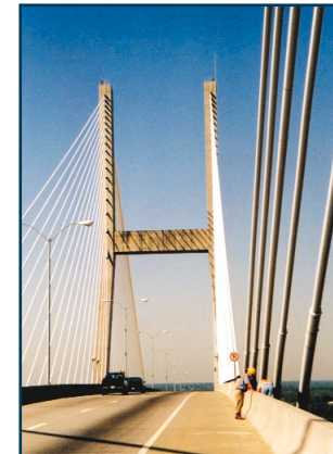
Engineer inspecting bridge cables
