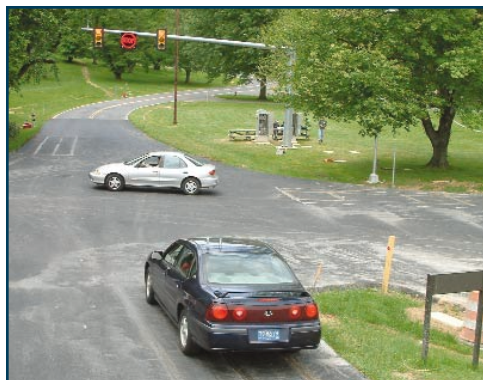
Intelligent Intersection at TFHRC.
