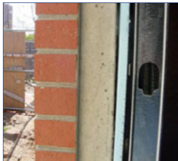
Wall construction consisted of 6 inch and 8 inch concrete panels, backed with half-inch expanded polystyrene foam insulation, steel framing, and R-11, faced, fiberglass wall cavity insulation.
