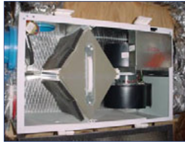
The Energy Recovery Ventilator tempers outdoor air before delivering it to heating and cooling equipment.
