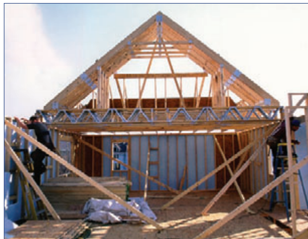
Advanced framing helps to save building materials and construction costs and create more room for insulation, making the house more energy efficient.
