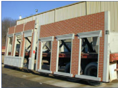
Precast panels helped to reduce labor costs and air leakage.
