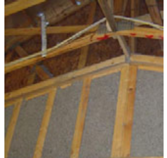
Blown-in wall insulation
