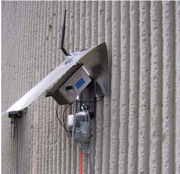
Figure 3. Close-up of an installed device
