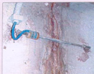
• Model 4420 Crackmeter installation
