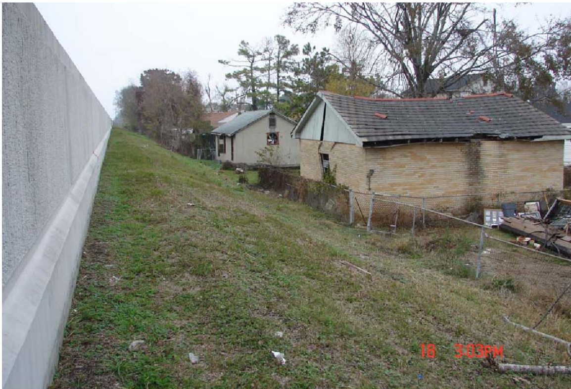
Figure 14. Photo of potential site #3, view looking north.
