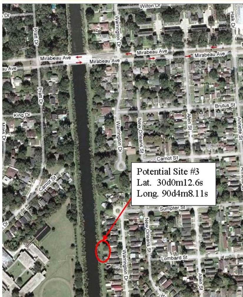
Figure 12. Aerial Photo of Potential Site #3.
